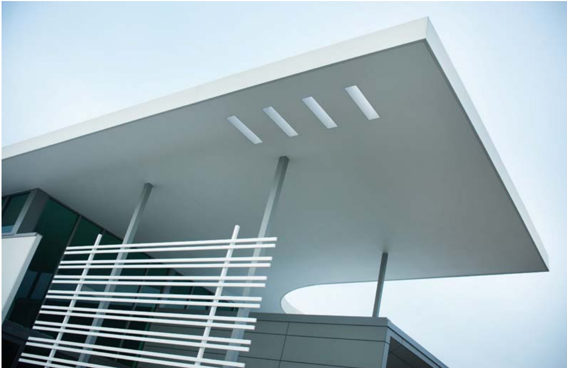
Entry awning – Department of Child Safety, Townsville, 2009
